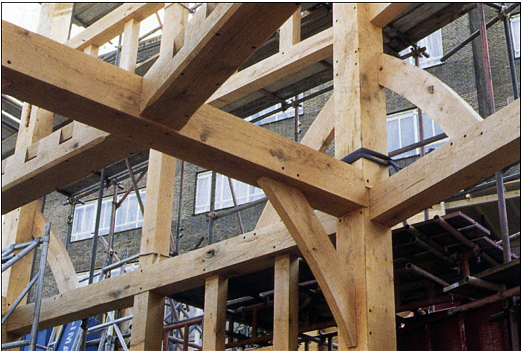
PLATE 9 Playhouse frame showing complex jointing.
